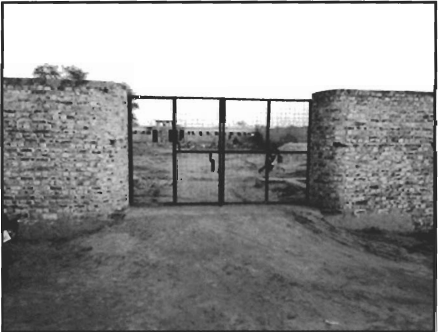
New Satsang hall under Construction ( 4 L.M. Anupgarh)
